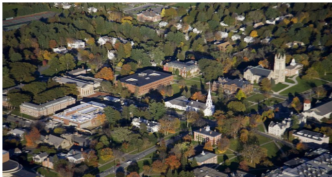
Figure 21 Williams College Aerial view
