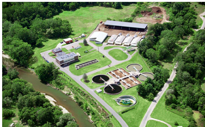
Figure 13 Hoosac Water Treatment Plant
