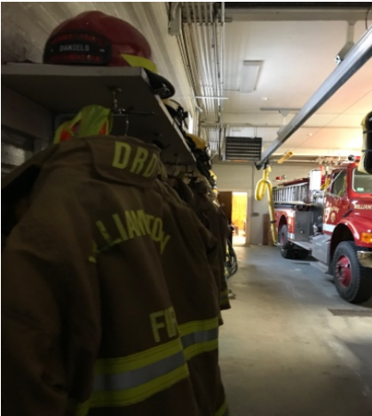
Figure 47 Fire Gear in Apparatus Bays
