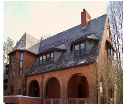
Figure 20 Williams College Main and Spring Street
