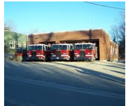
Figure 5 Williamstown Fire Station
