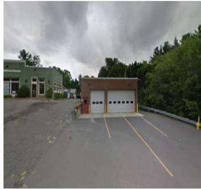
Figure 3 Williamstown Fire Station 34 Water Street Williamstown Mass
