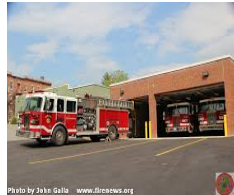
Figure 42 Modern Fire Apparatus at Water Street Fire Station
